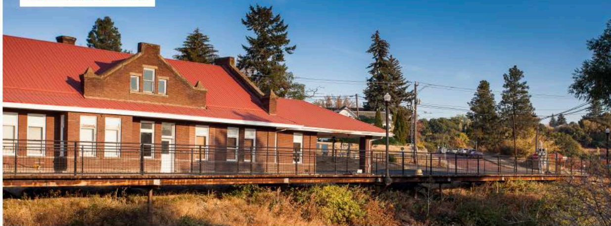
Afternoon sunlight on Northern Pacific Depot's newly visible west side, with view up to College Hill through the brick roads.
